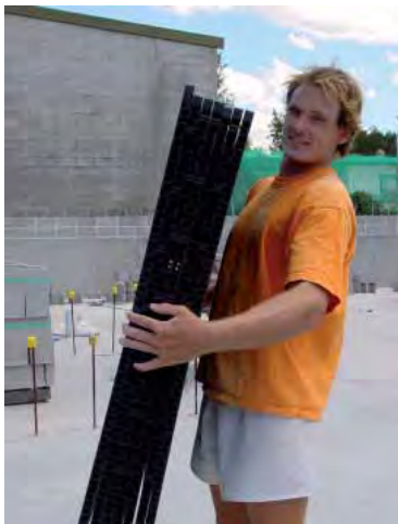
On site labour easily handles 10 m 2 of lightweight pre-assembled panels.
