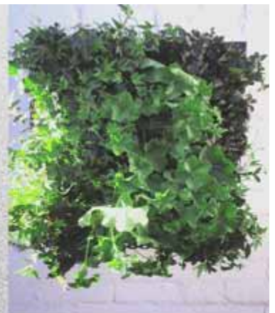
Modules containing plants are mechanically anchored onto walls
