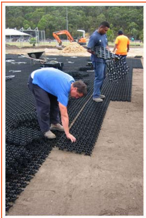
TurfPave® being installed at the Sydney
