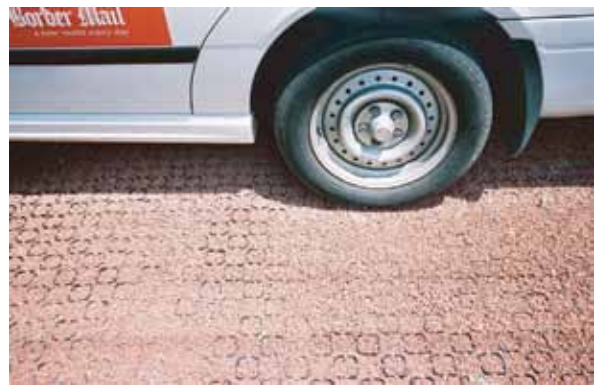
Albury Council in NSW installed TurfPave to stabilize scoria on verge parking areas.
