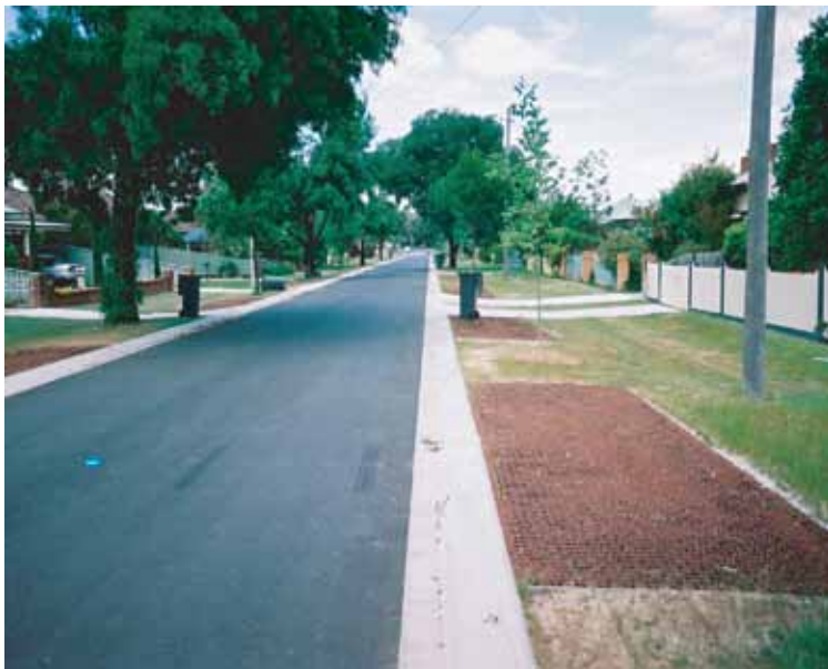
Albury Council in NSW installed TurfPave to stabilize scoria on verge parking areas.
