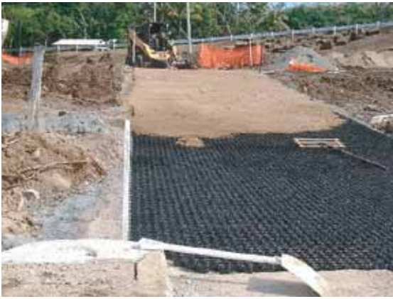
TurfPave stabilizes salt tolerant paspalum on boat ramps at Airlie Beach on the Whitsundays in Queensland.
