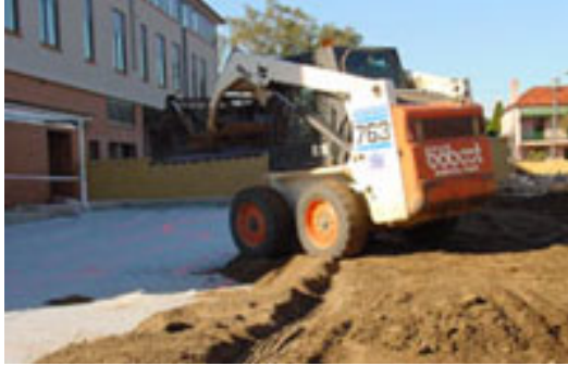
VersiCell, when covered with soil, withstands the weight of heavy equipment.
