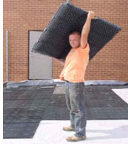
An installer easily carries 6m 2 of interlocking lightweight pre-assembled panels.
