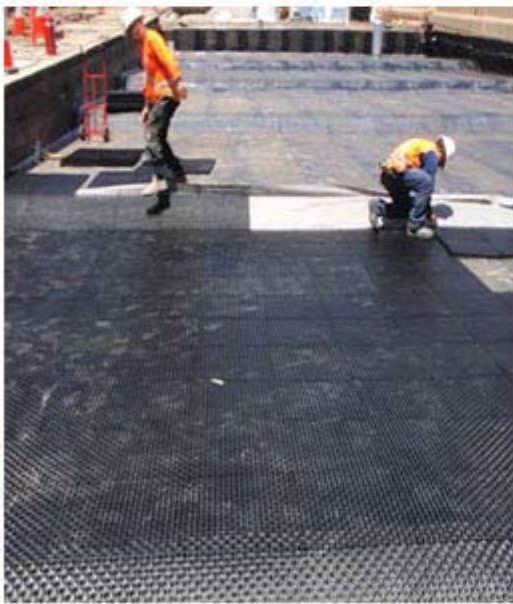
Specified and installed by Eptec Pty Ltd. ,VersiFlex conforms to uneven surfaces and ensures efficient drainage under high weight bearing trafficable access roads at Central Railway Station Sydney.
