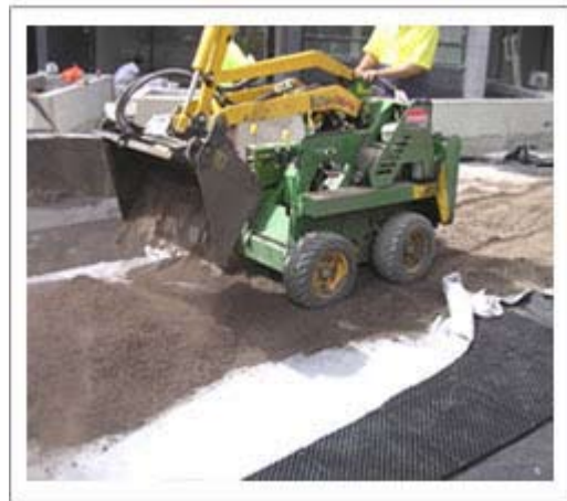
VersiFlex will withstand the weight of mechanical equipment
