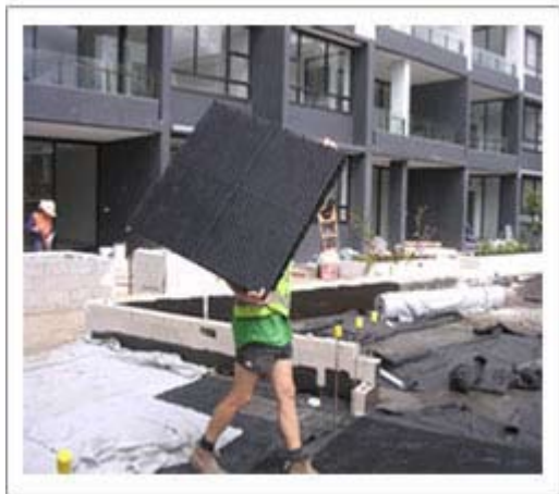
Large pre-assembled VersiFlex panels are lightweight and rapidly installed
