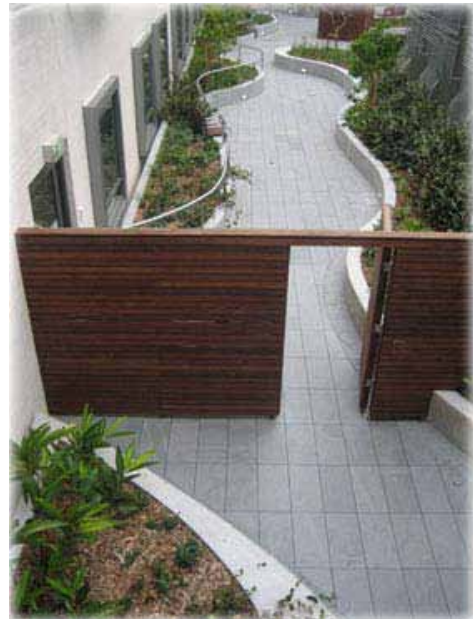
VersiPave®GP allows easy access to waterproofing membranes and services at the Burger Retirement Centre at Randwick in Sydney
