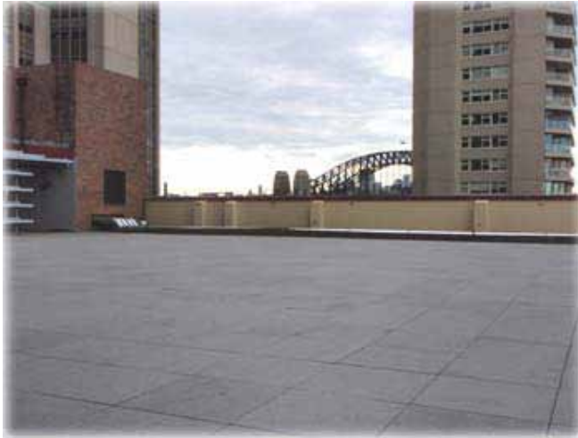
The 1,200m 2 free draining rooftop of Transport House in Sydney (above), with pavers supported on VersiPave®GP positioned on insulation board (below).
