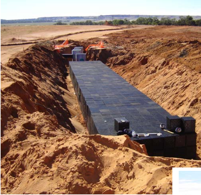
A large VersiTank installation in Geraldton Western Australia, supplied by Geofabrics Australasia Pty Ltd., acts as an underground infiltration system for storm water run-off from an industrial estate.
